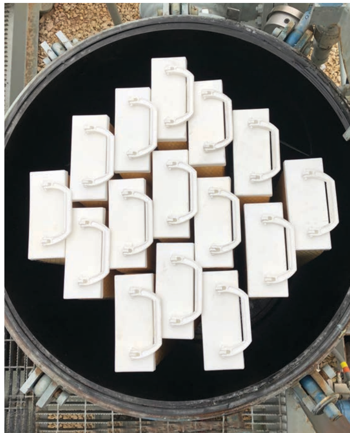
Invicta™ cartridges installed on new guideposts
